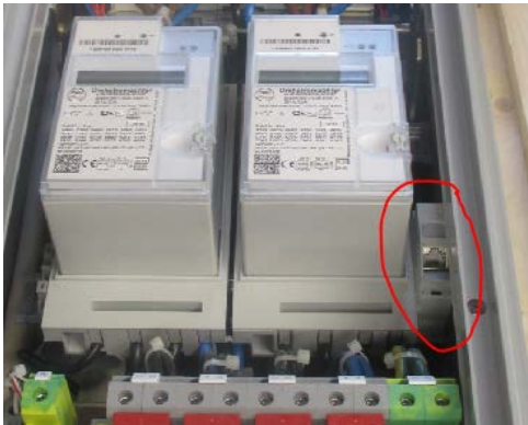
Abb. 1: Ethernetbuchse (RJ45)
